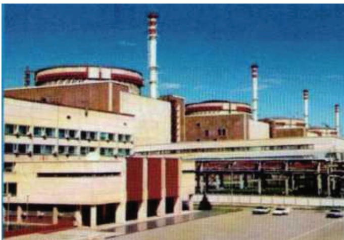
Balakovsky Nuclear Power Station
