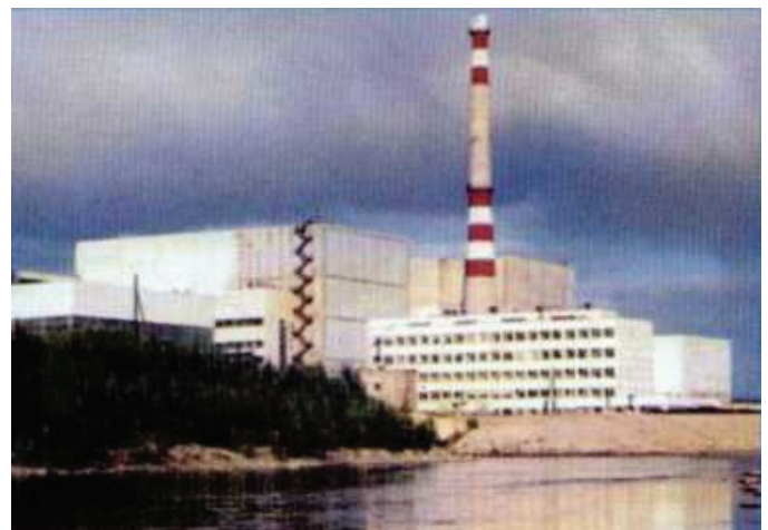
Kole Nuclear Power Station
