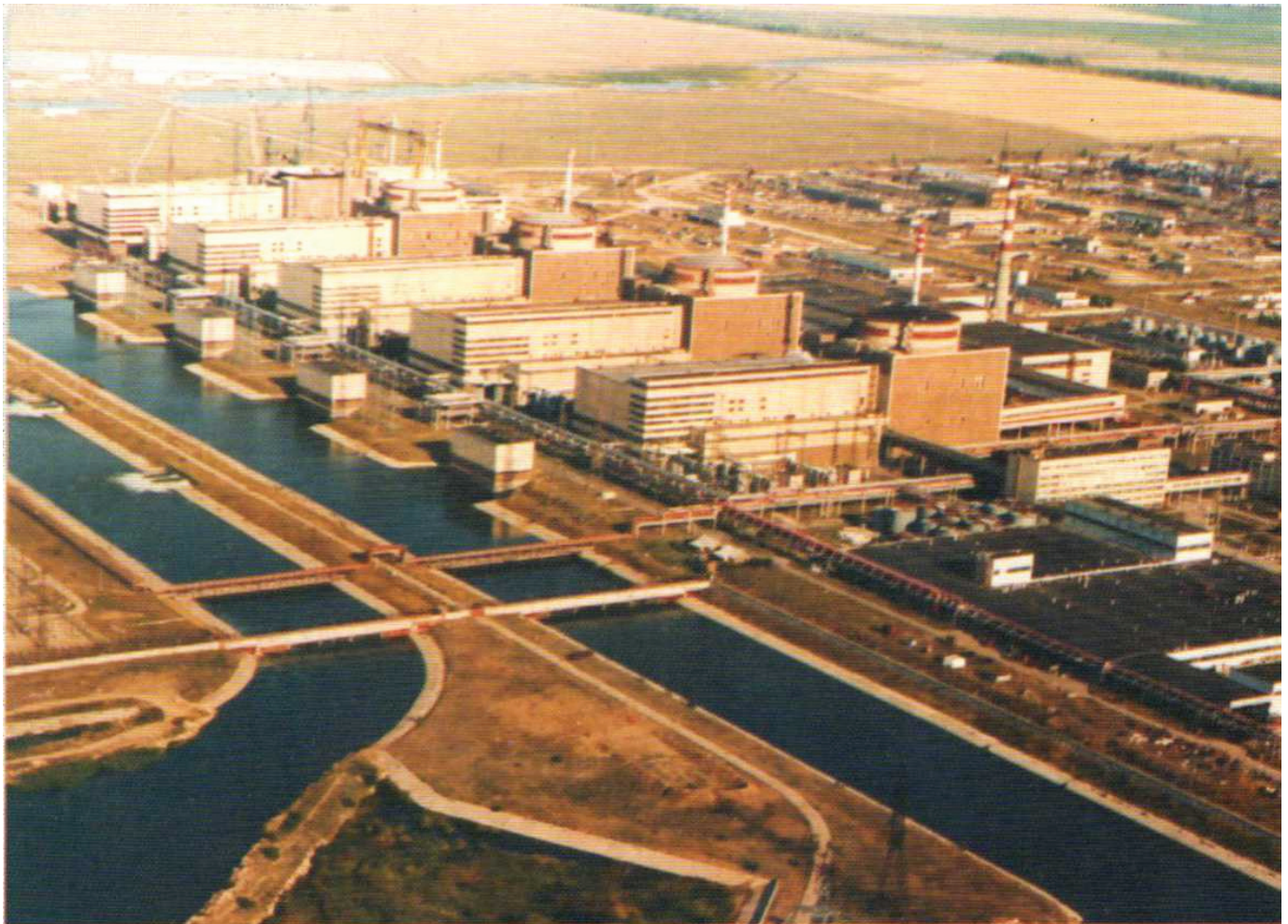
Balakovskaya nuclear power station
