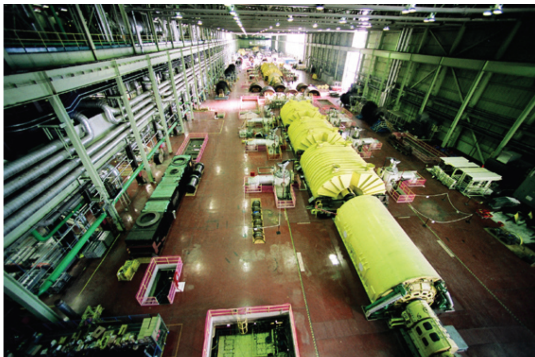
Balakovskaya nuclear power station
