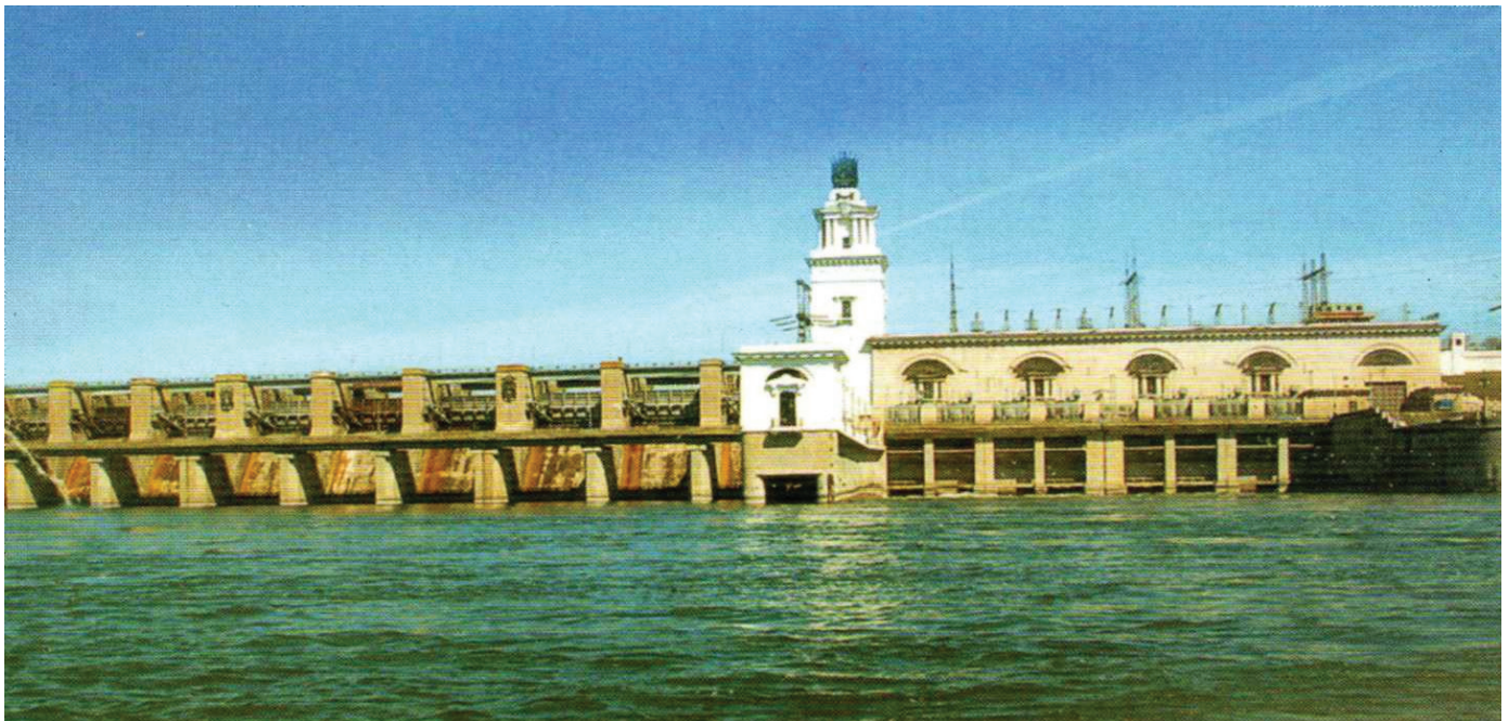
Zimlyanskaya hydroelectric power station
