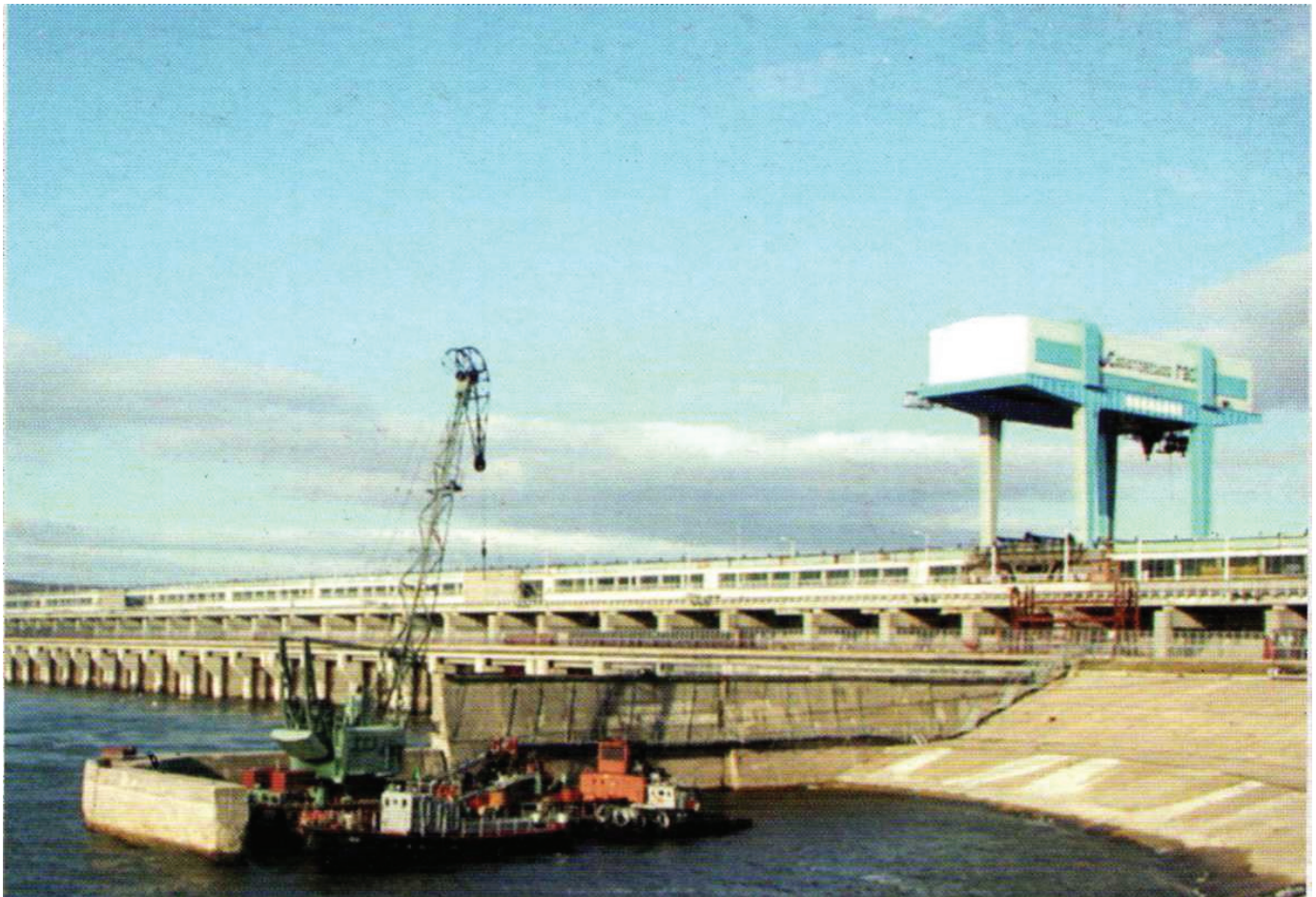
Saratovskaya hydroelectric power station
