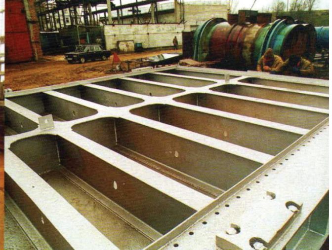
Strengthening assembling Area. Lock reconstruction of Saratovsk irrigation canal
