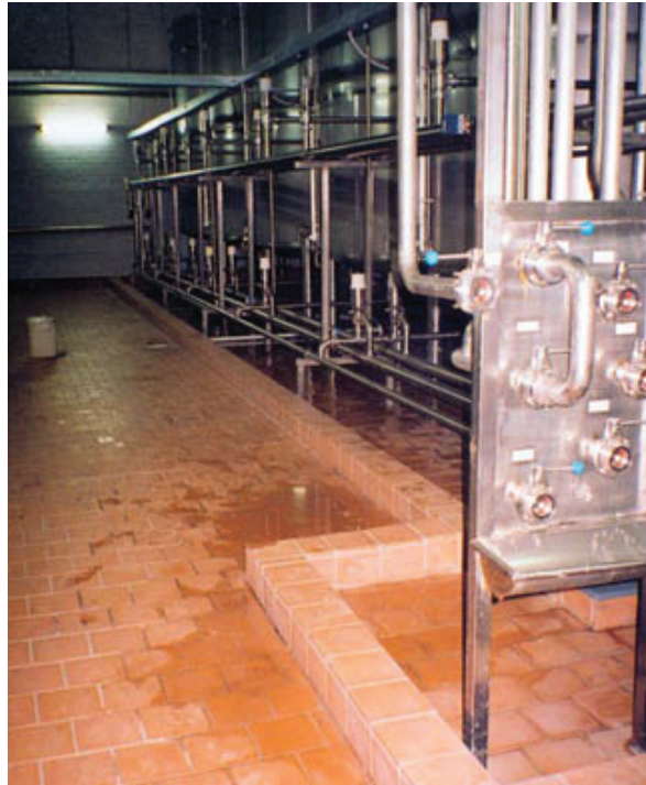
Floor made of acid-proof bricks
