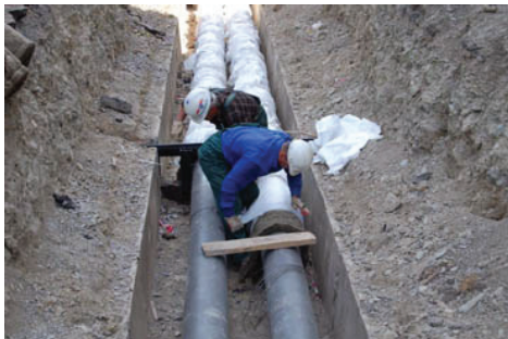
Heating main roads assembling, metal constructions
