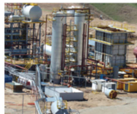
Oxidation columns made from high-temperature steel
