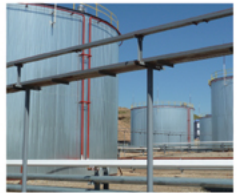
Raw materials tanks and ready product tanks equipped with a heating system to prevent solidification of products, automated filling control, insulated.
