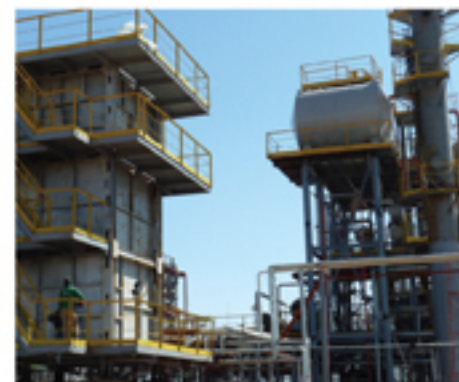
Furnaces made from special high-temperature steel, brick lining with asbestos for temperatures up to 1000 C
